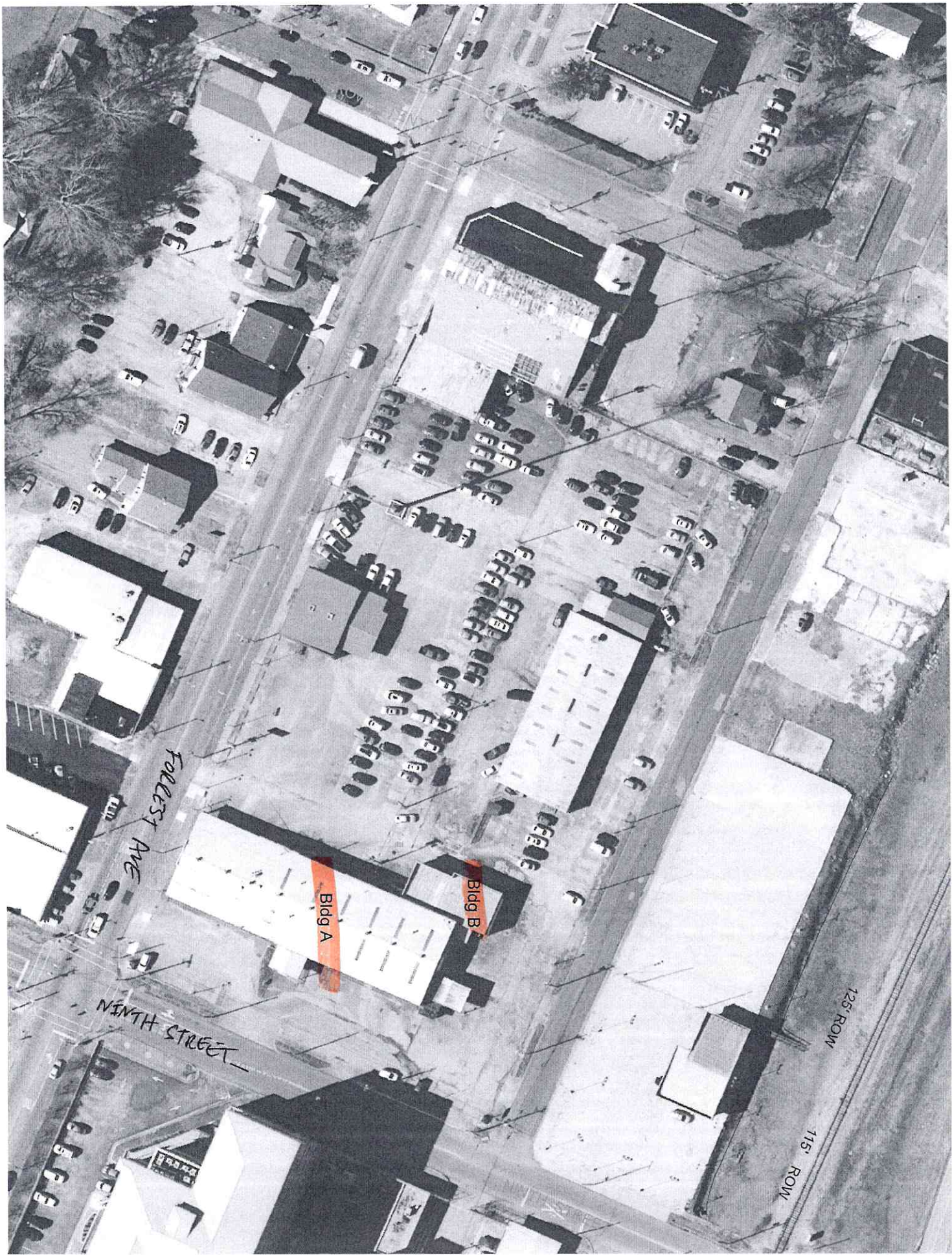
All other attached structures, not in contract.
